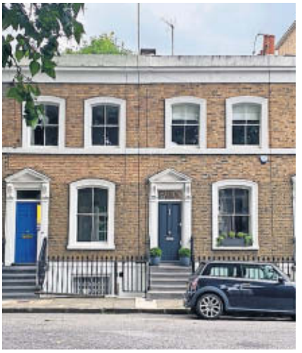
► Keval Khuroya would like to add a mansard roof to his terraced house in Islington, right, similar to ones in nearby streets, below right
